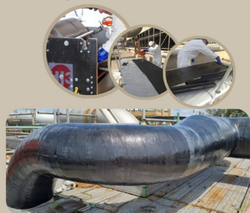
Figure 3: Field-saturated, field-cured composite repair system
