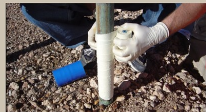
Figure 2: Pre-saturated, field-cured composite repair system
