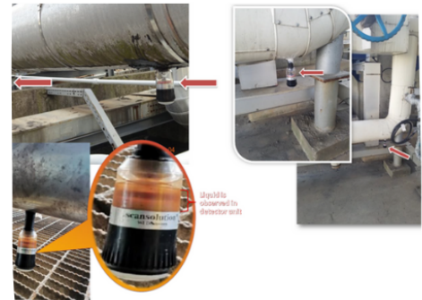
Figure 6: WI Discovery Leakage Detector with “photos” of installed locations.
