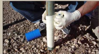
Figure 2: Pre-saturated, field-cured composite repair system
