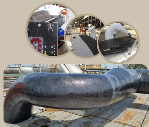
Figure 3: Field-saturated, field-cured composite repair system
