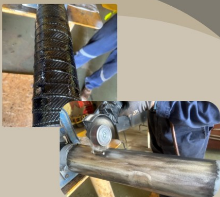
Figure 7: Installer qualification hand on installation training
