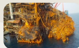
Figure 9: Collapse of offshore platform due to fire and explosion
